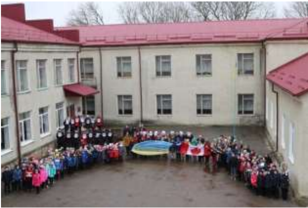
Horynka School with new roof
